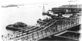
Northern Avenue Bridge, The Bell House, Pier 1 — South Boston.
