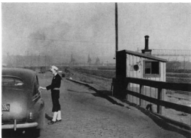
Ramp at Mystic. What memories to be recalled of hours within and without this old shack! Scope of Mystic post was from Snyder Fuel at Pier 45 (extreme left) to scrap and coal piles on river (far right) to harborfront Piers 46-47, 48-49-50.
