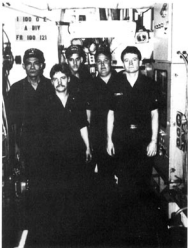
"THE BOILER ROOM GANG" L to R MK1 Juhin, MKCM Tobols, FA Kuypers, FN Bolan, FN Amley
