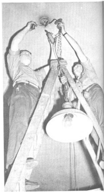
Two electricians repair fixture.
