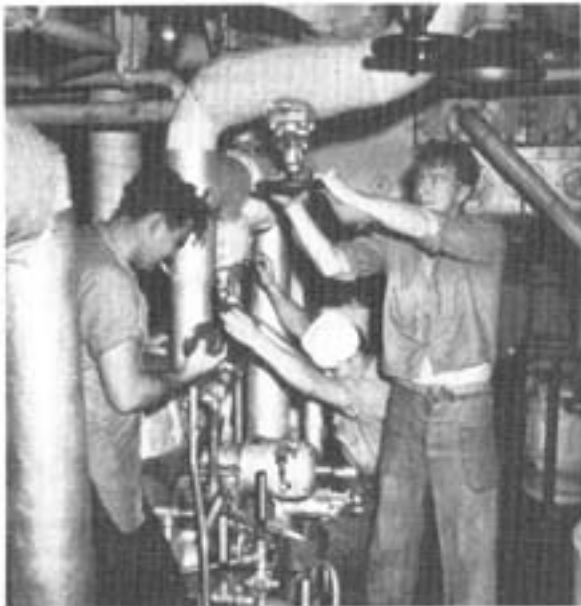
SERVICING MAIN PUMPS
