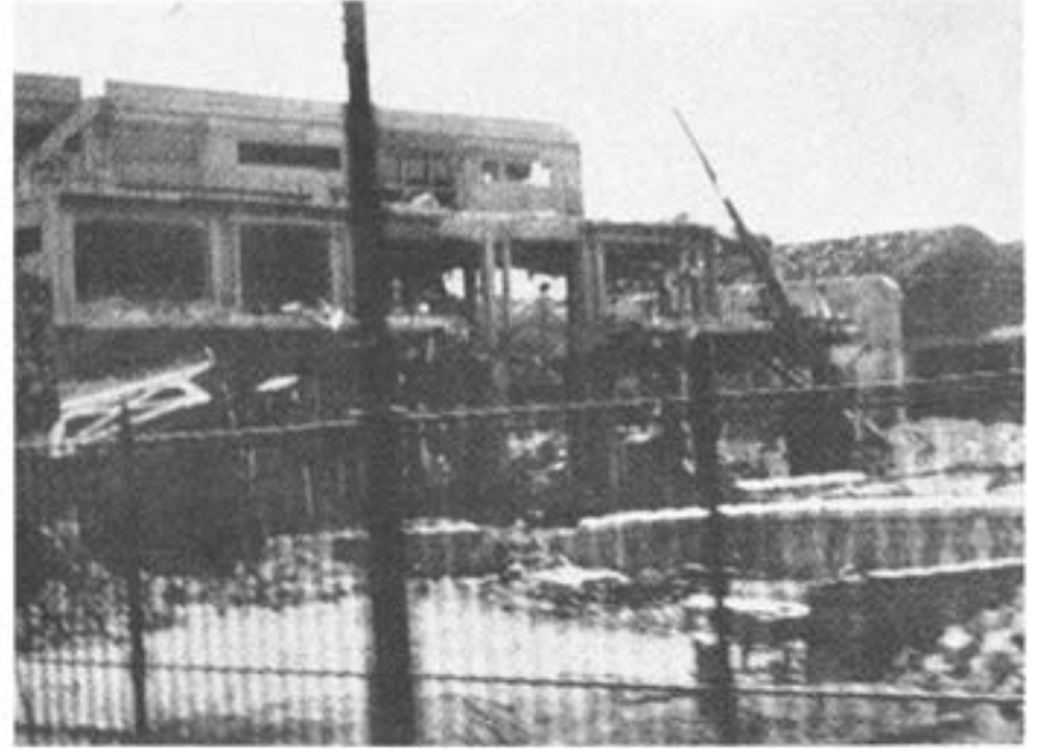
BOMB DAMAGE — MARSEILLE
