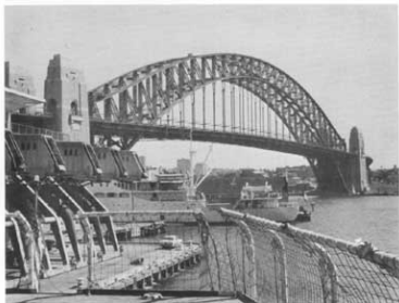
Outstanding landmark of city; Sydney Harbor Bridge.
