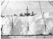
carried to edge of barrier and planted in position. Blast (bottom) causes ice to fall away into sea. Black marks (right bottom) show where charges drove down barrier.
