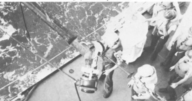
Standing by to hook up fuel hose
