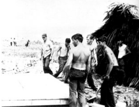
The floor being put in place for the new dispensary.
