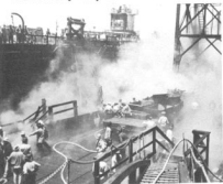
Fire nearly out, smoke turns white
