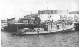
Early picture of Station #2 shows 57005-F
